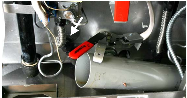
Figure 1: Drain tubes blocked by cabinet uprights must be rotated downward
